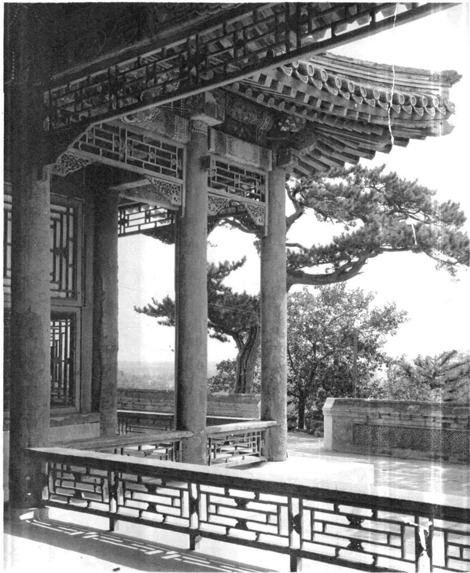
Plate 62. Pavilion-gallery at the New Summer Palace, provided with ornamental balustrades and lambrequins. The latter, resting on brackets, form a continuation of the decorated beams under the eaves.
